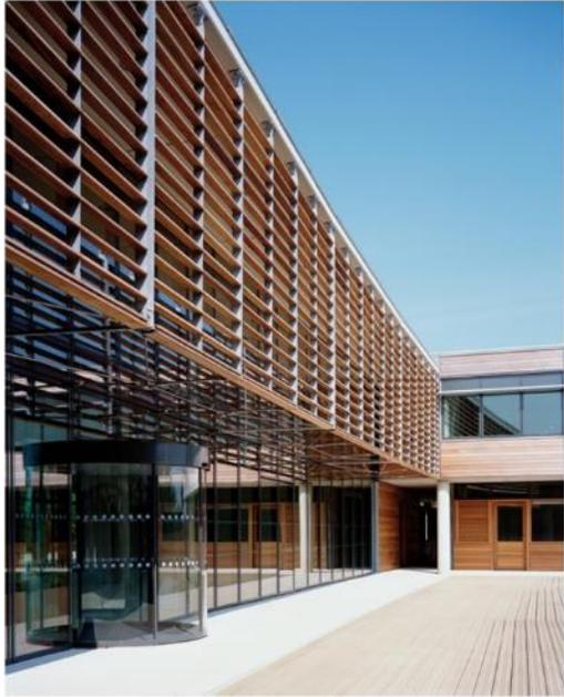
Solar shading to the entrance building will be a vertical array of horizontal timber aerofoil section fins
