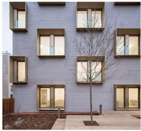
Deeply recessed windows with projecting linings to CSB first floor laboratories
