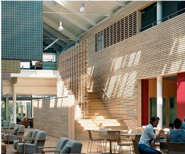
The interior of the entrance building will use timber extensively on walls to form acoustic panels and bring warmth to the space. The extensive glazing to the external walls will mean that this will be clearly visible as you approach the building
