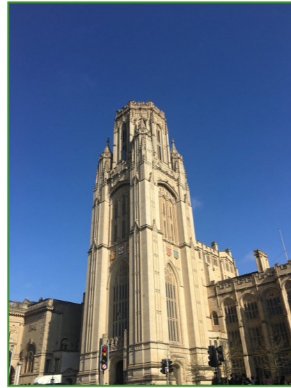
The Wills Memorial Building Photo: Stephanie Smith
