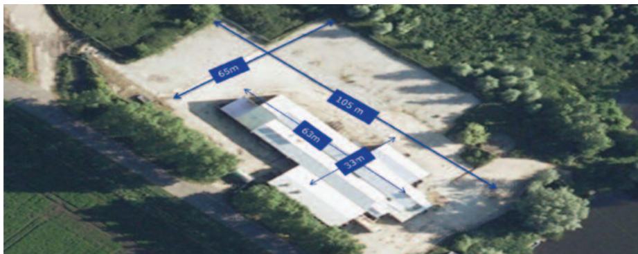
The site prior to construction of the new NIAB field research facility
