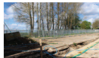
Additional fencing to isolate the ditch during construction work
